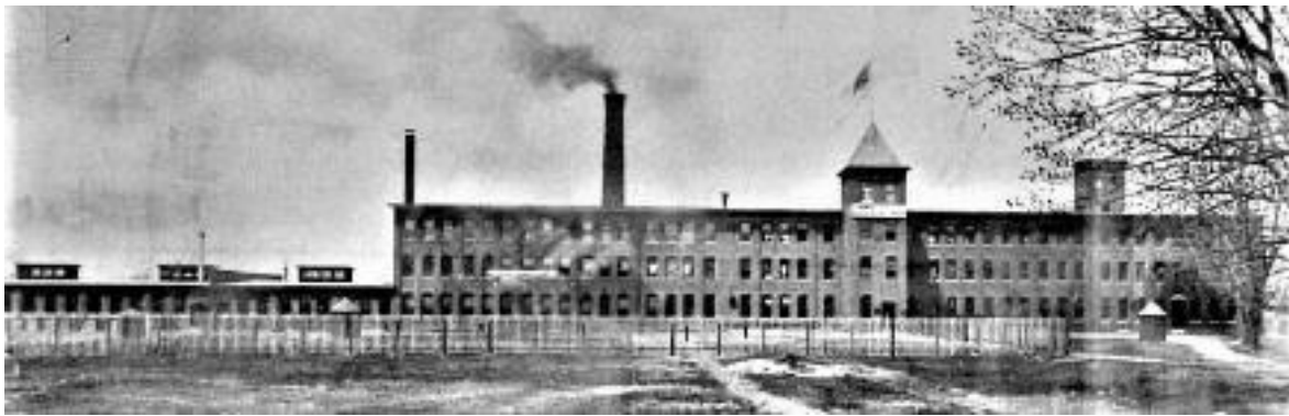
A photograph of the plant, date unknown
